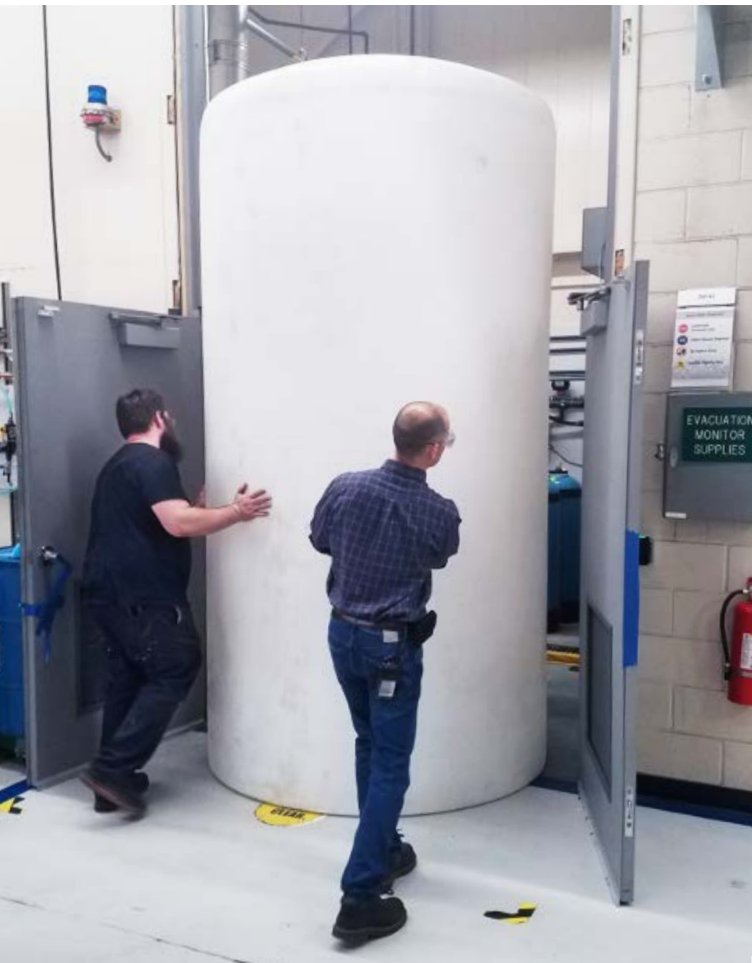
New 1,500gal neutralization tank.
