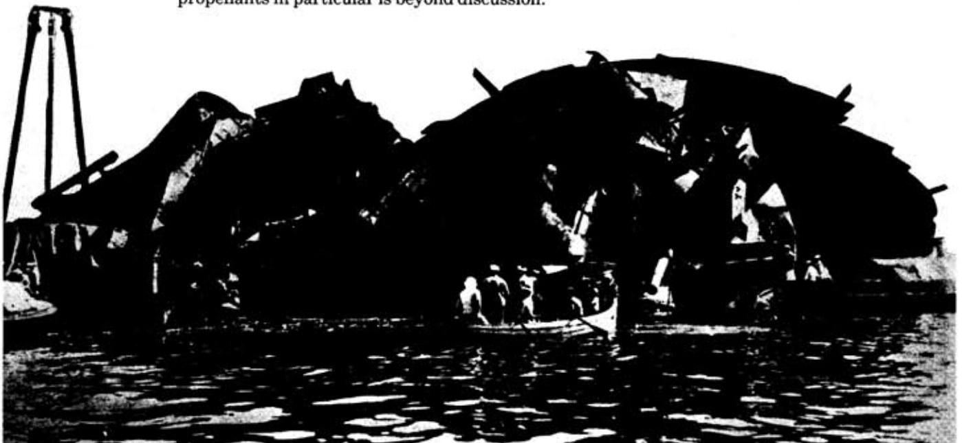
Fig 1. The French battleship "Liberté" destroyed by a propellant explosion in 1911.
