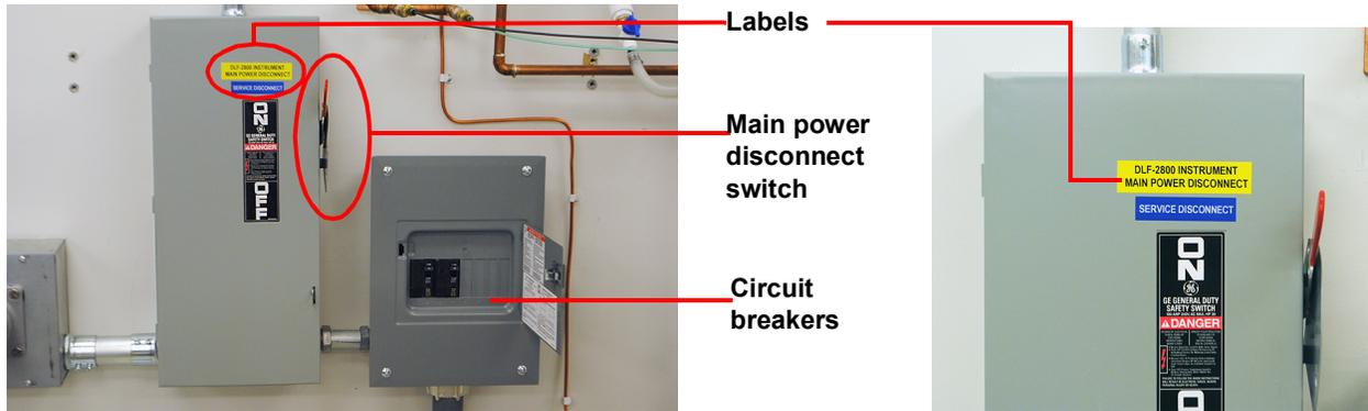
**Figure 7** Left: Main power disconnect switch and circuit breakers; Right: Supplied label.
